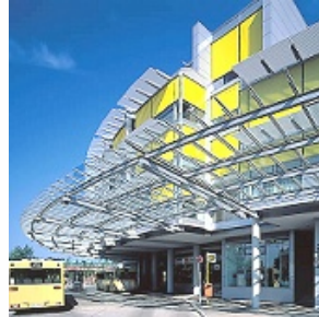
Building 7 with Bus Depot
